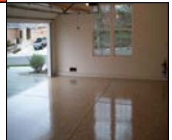
Garage Floor showing the 1 coat high build
