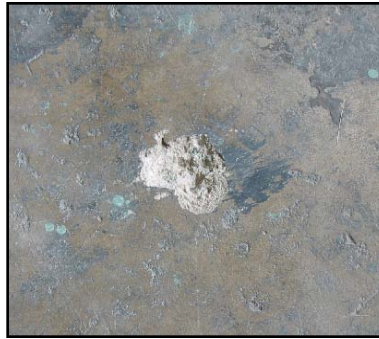
Spalled Concrete
